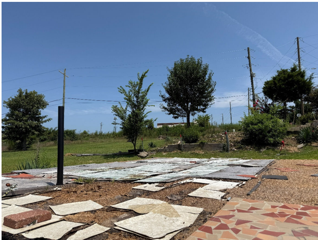
Photograph 5: A view of the remaining floor covering of the house.
