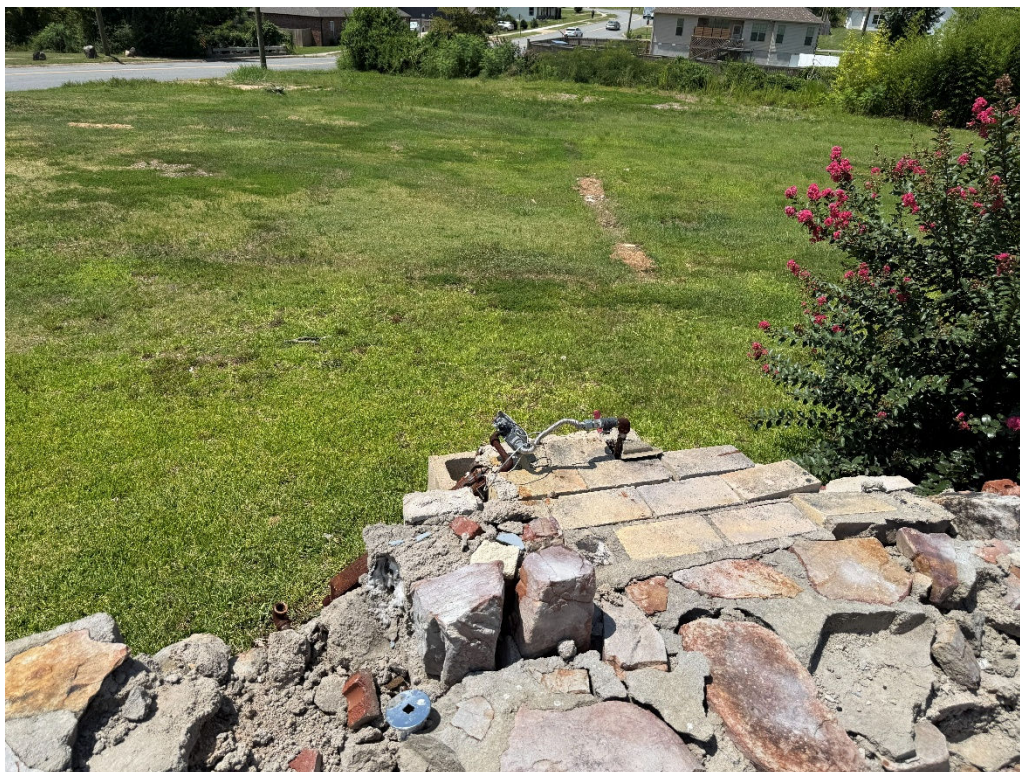
Photograph 6: A view of a natural gas pipe.
