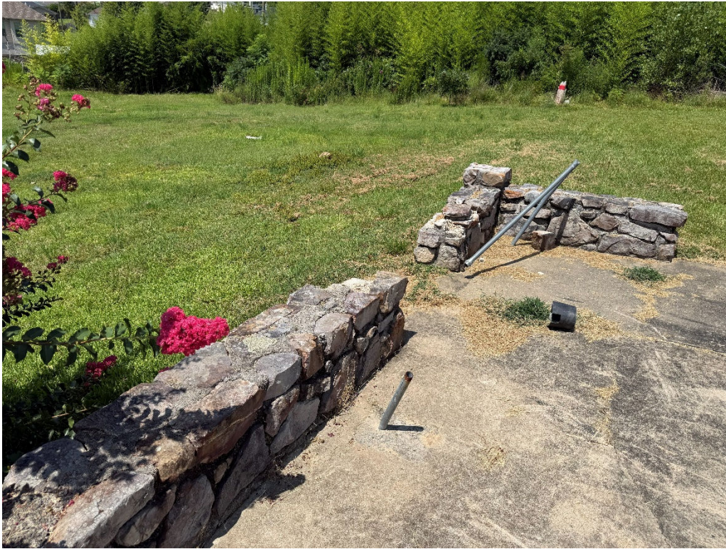
Photograph 3: A view pipes extending out of the slab.
