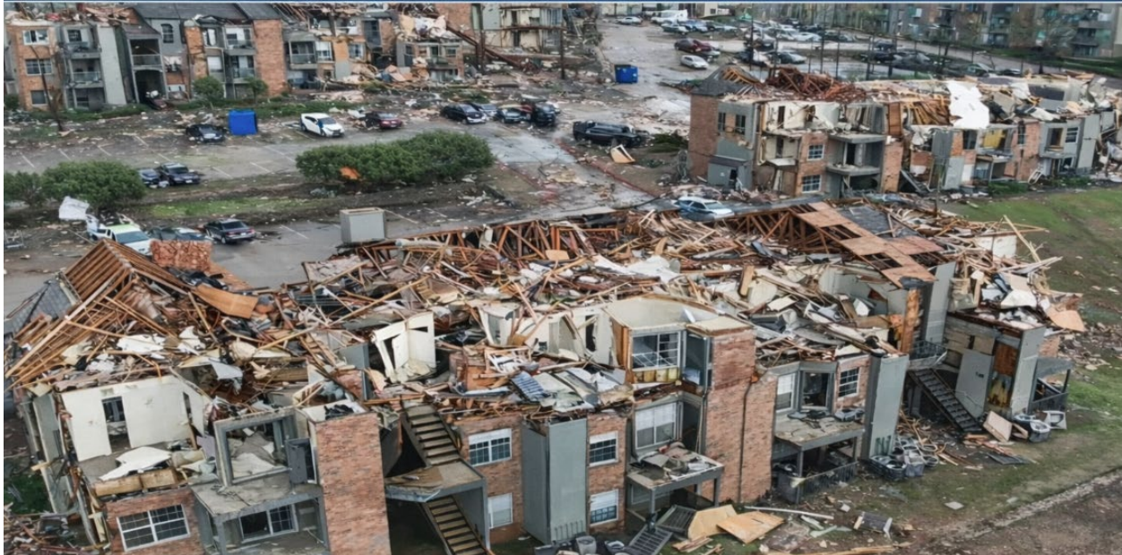
Figure 1. Housing Damage Conditions Following DR-4698
