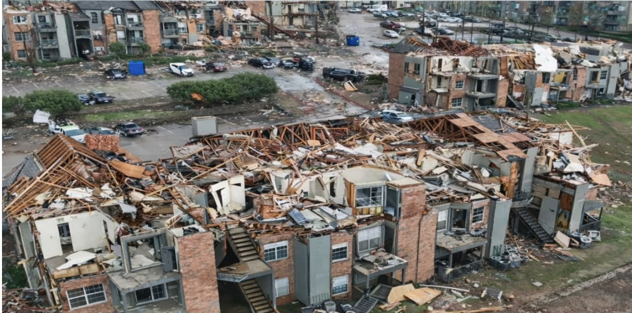
Figure 1. Housing Damage Conditions Following DR-4698
