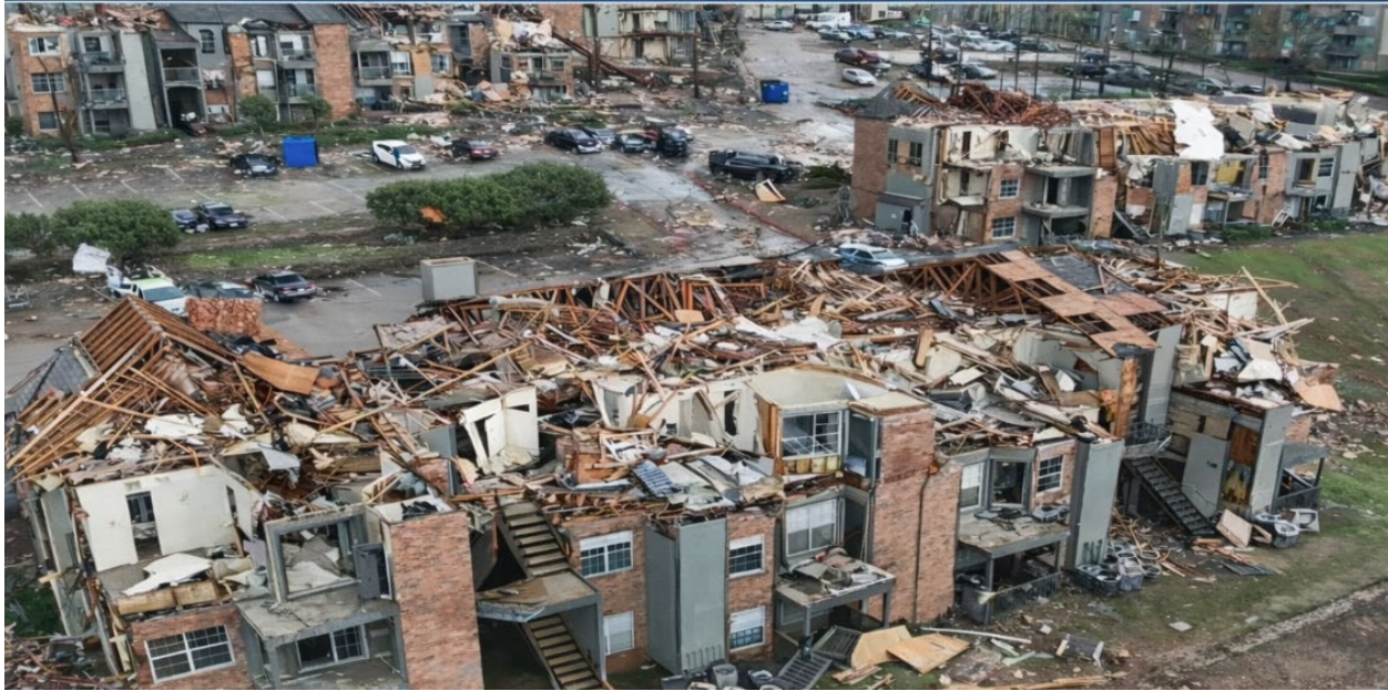
Figure 1. Housing Damage Conditions Following DR - 4698
