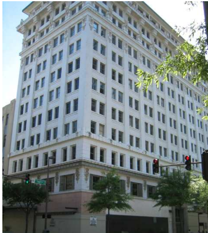
Though the first floor façade has been altered, the State Bank Building (known today as the Boyle Building) at Fifth and Main still looks much as it did when it was completed in 1909.
