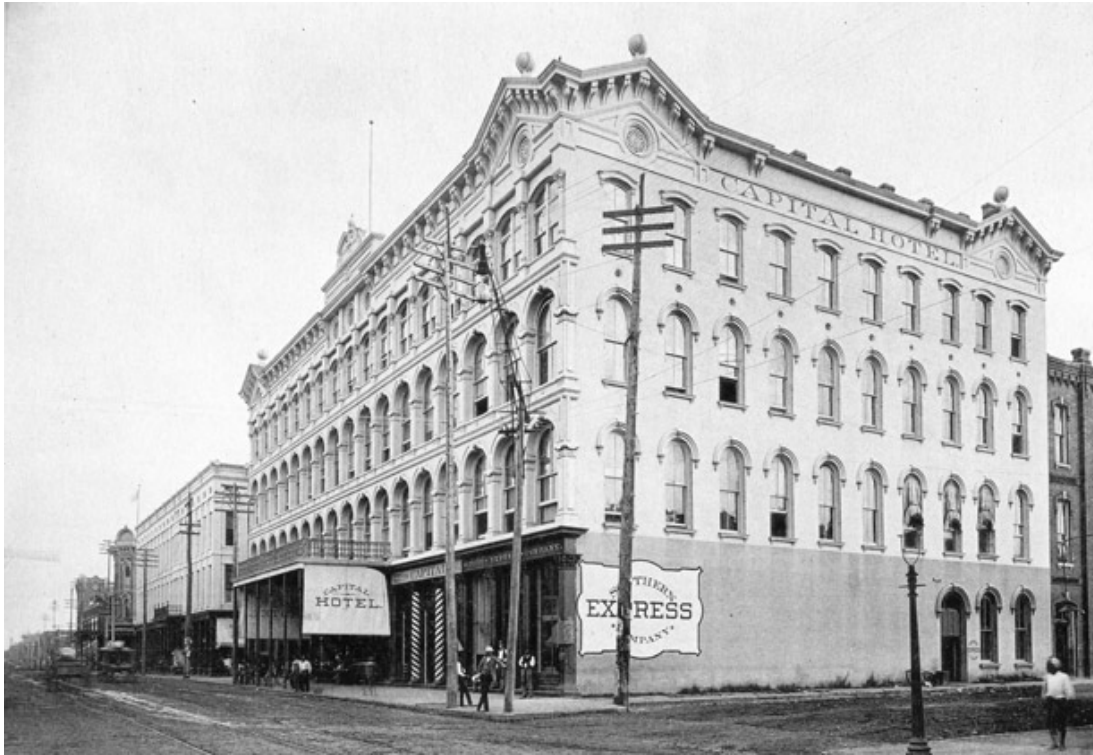
The Capital Hotel was built on Markham Street in 1872. One of the hotel's most notable features is its prefabricated cast-iron façade. (photo ca. 1892)
