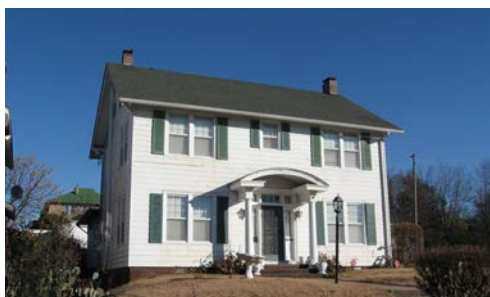
The Historic Preservation Task Force of 1996 stressed the need for completion of survey and National Register efforts for areas such as south of Roosevelt Road (2723 S. Ringo Street).
