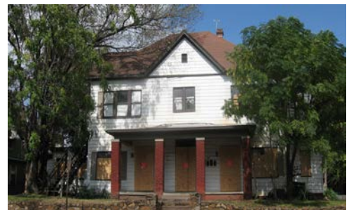
Demolition by neglect provisions would require owners of vacant properties to maintain houses to minimum standards (420 E. 9 th Street).
