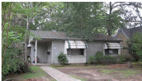
At 1302 Tyler Street is a Lustron House which was built with an exterior of steel porcelain panels.
