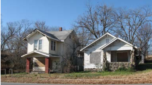
Abandoned houses in the 1600 block of S. Woodrow.
