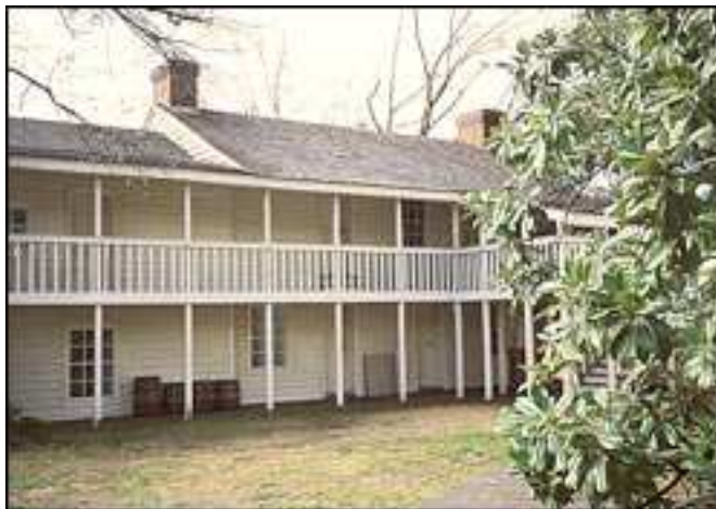
The Hinderliter Grog Shop as it appears today as part of Historic Arkansas Museum. Originally log, the building was later covered with frame siding.
