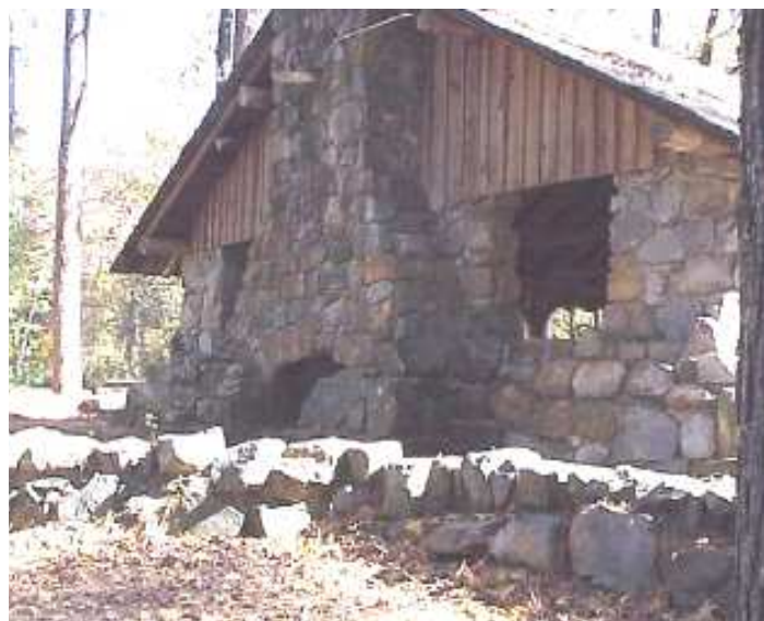
The stone and log construction of CCC pavilions at Boyle Park is typical of the federal park projects of the era.
