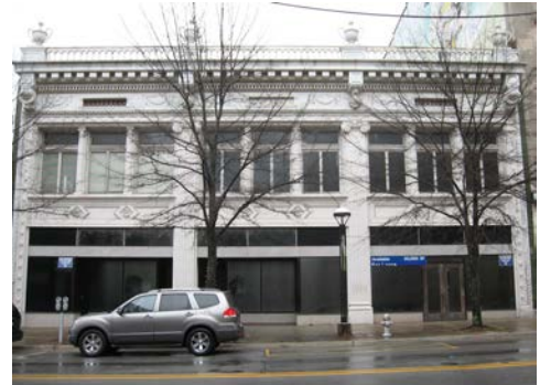
The Rose Building at 307-311 S. Main Street was an early federal tax certification project.
