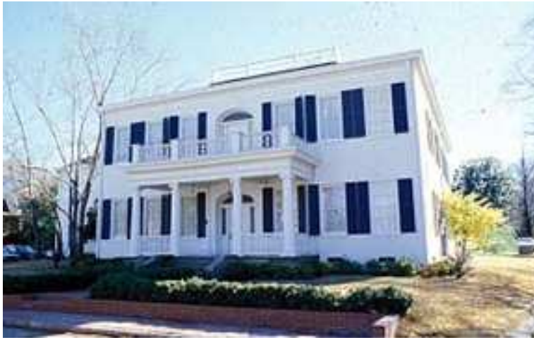
The Absalom Fowler House built in 1840 has Federal elements but echoes the Greek Revival style with Ionic columns supporting the portico.
