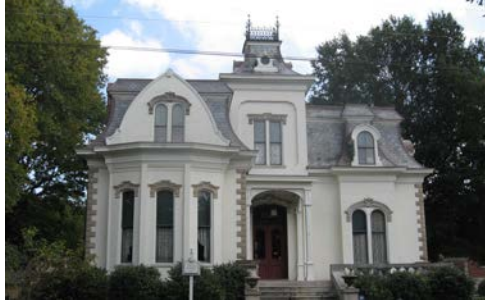
This Second Empire style dwelling at 1321 Scott Street in MacArthur Park is the Villa Marre and reflects the rich legacy of the city's older neighborhoods.
