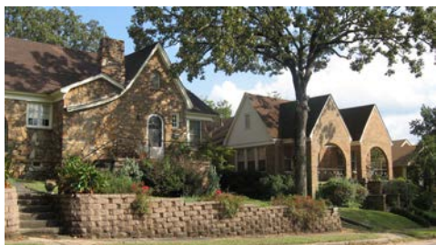
Many of the city's most desirable neighborhoods are located within National Register Historic Districts, such as the 400 Block of Pearl Avenue in the Capitol View Historic District.
