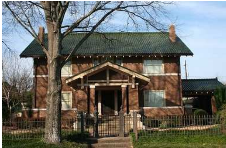
The Keith House built in 1912 on Broadway is one of the city's best examples of Craftsman architecture. Its low-pitched roof with exposed rafter ends, decorative braces under the eaves and broad porch roof supported by square columns are all Craftsman characteristics.
