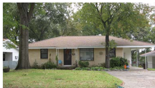
At 10 Berkshire Drive is a standardized plan hipped roof Ranch style dwelling with an attached open carport.
