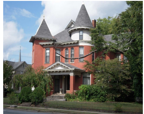
Because Queen Anne houses such as this one in MacArthur Park can accommodate more than one dwelling unit while retaining their historic integrity, the City’s Future Land Use Plan designation of Low Density Residential is compatible with this historic neighborhood.
