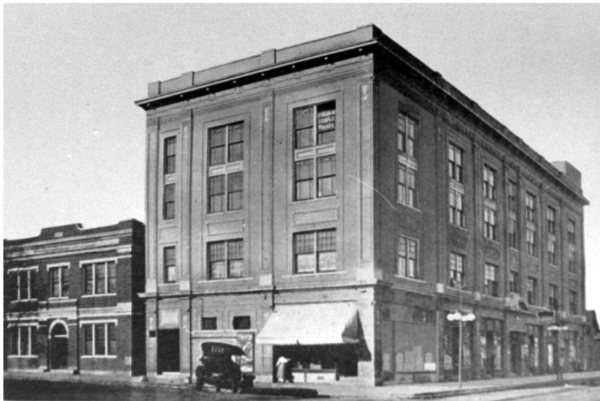
Built in 1911, the headquarters of the Mosaic Templars of America was one of the most significant buildings in Little Rock's African American community during the early-20 th century. Founded in 1883, the fraternal organization provided insurance and other services to African Americans in 26 states. (Photo is from 1924).
