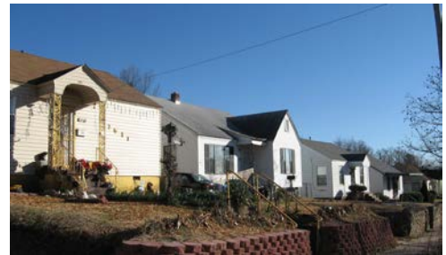
Future survey efforts should concentrate on neighborhoods, such as South End, where there are large numbers of pre-1945 dwellings (2600 block of S. Cross Street).
