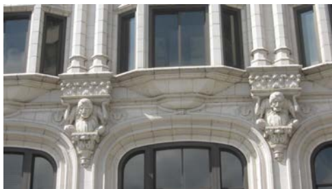
Downtown Little Rock contains an impressive collection of late 19 th and early 20 th century commercial buildings (212 Center Street).
