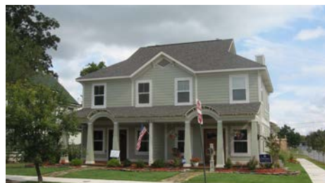
Conservation zoning or limited historic ordinance districts would ensure that new construction was compatible with adjacent historic buildings. This new dwelling was subject to design review in the MacArthur Park Historic District (1421 Cumberland Street).
