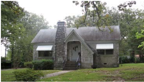
This Tudor Revival dwelling was built at 1301 Taylor Street with an exterior of stone veneer.
