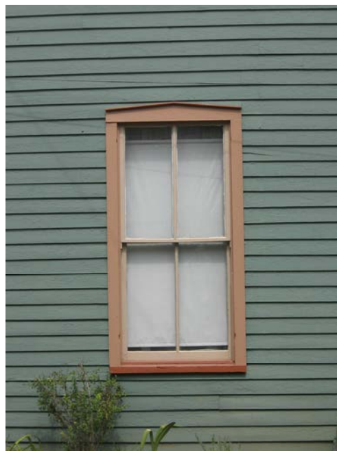
Preserving and maintaining original wood windows is often more cost effective than replacement with new window units.
