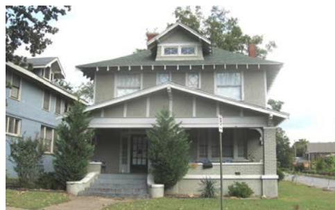
The 2006 Downtown Plan addressed the need to increase rehabilitation and home ownership in neighborhoods such as Dunbar (2321 S. Ringo Street).
