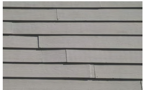
Do not use replacement materials that do not match the character of the original wood, as this can lead to architectural failures. © Scribeware
