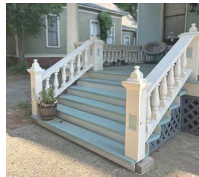
Wood steps match the porch floor at 514 E 8th St.
