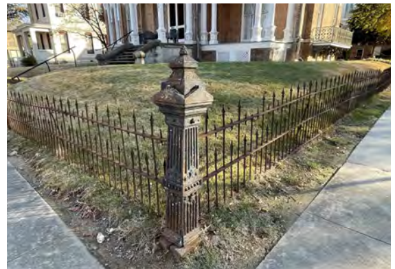
Retain and preserve historic fences. (301 E. 7th St.)
