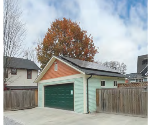
A side gable garage roof with solar panels, 1410 S. Rock St.
