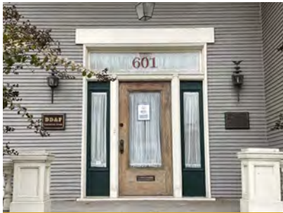
Historic door with sidelights and transom at 601 S Rock St., Nash House
