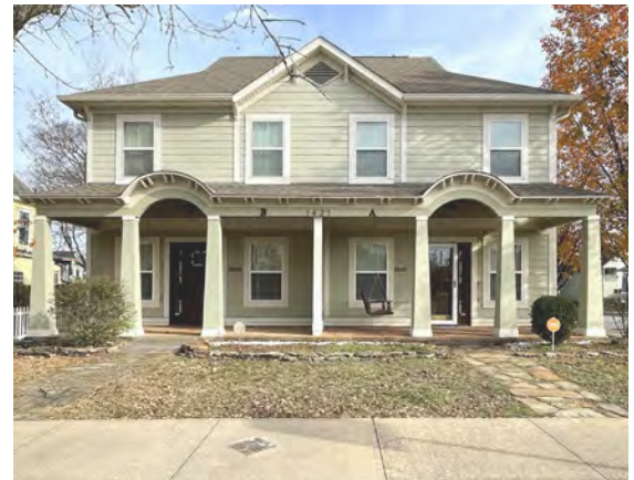
New roof areas should be compatible with the roof forms, types, shapes, and pitches found within the area of influence, 1421 Cumberland St. ✓
