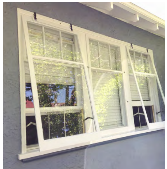
Add storm windows as a second barrier against the elements and air infiltration. © Spenser Works
