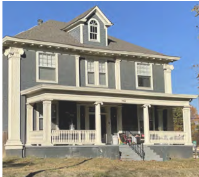
A Prominent dormer at Power House at 1402 S. Commerce St.
