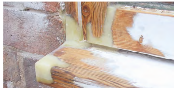
For small areas of deterioration, repair wood using commercial wood epoxies. © Repair Care Co UK
