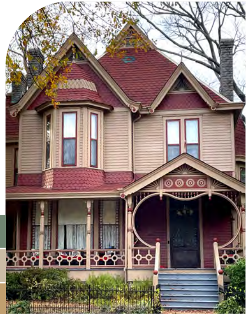
Hanger House at 1010 S. Scott St.
