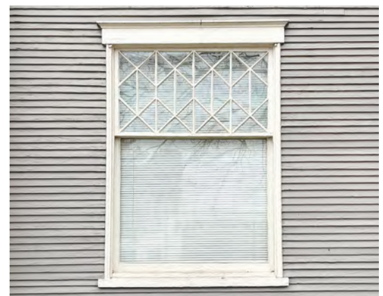
Decorative upper sash in historic wood double-hung window, 601 S Rock St.
