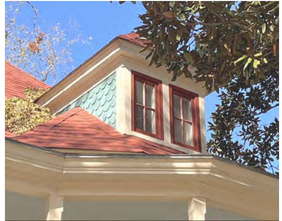
Well maintained dormer, 904 S Rock St.
