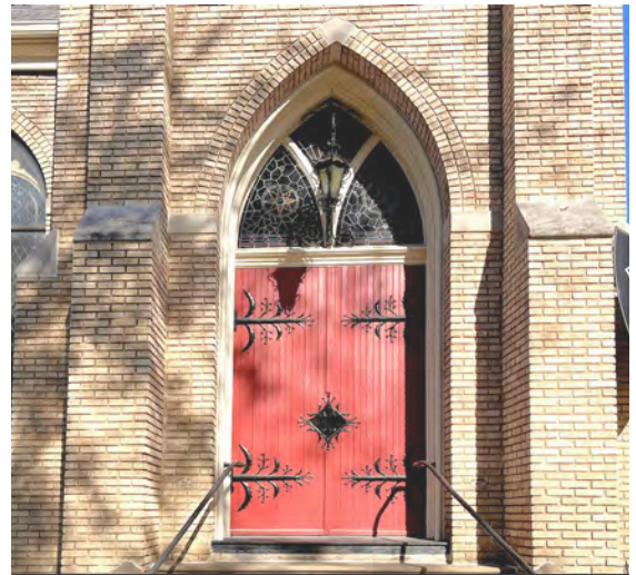
Preserve character-defining historic hardware in its original location even if it is no longer functional, 318 E. 8th St.
