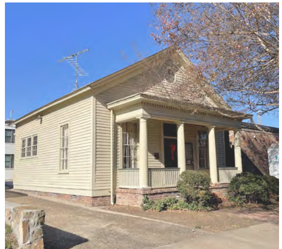
Preserve and maintain historic foundation materials that are in good condition, 610 S Rock St.
