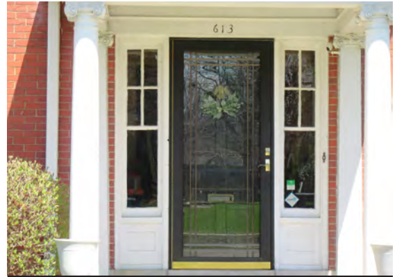
Add a storm door as a second full barrier against the elements.
