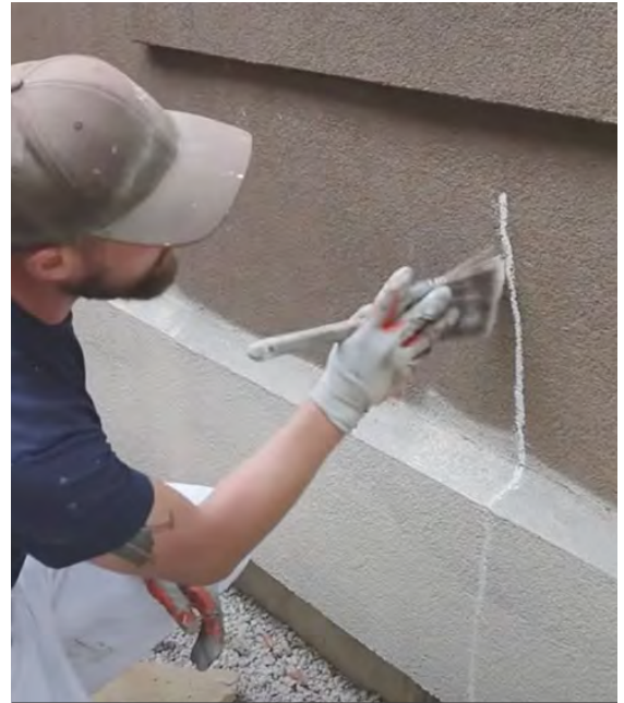
Use paint or limewash to repair small cracks in historic stucco. © Tape University
