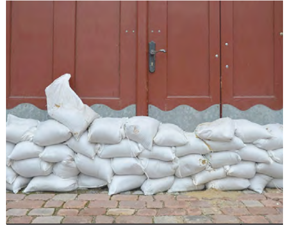
Implement temporary measures including sandbagging to address the potential for, and impacts of, flooding. © CallMSI
