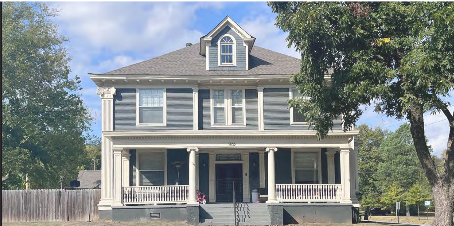
Powers House at 1402 Commerce St. restored exterior walls post fire.
