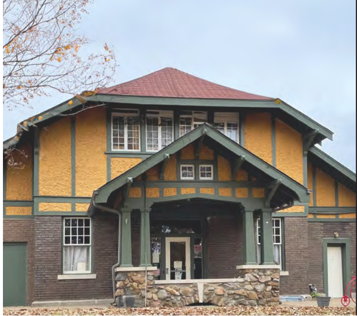
Fire Station No. 2 at 1201 S Commerce St.
