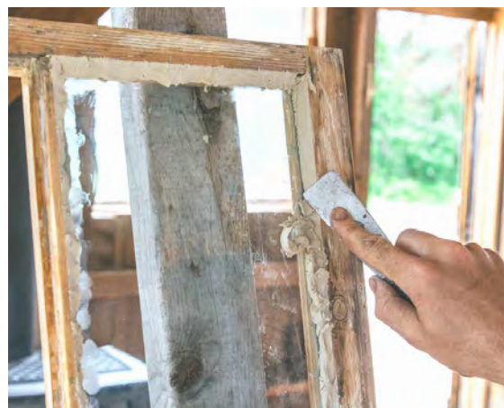
Remove damaged glazing and replace glazing putty. © Mortise and Tenon Magazine
