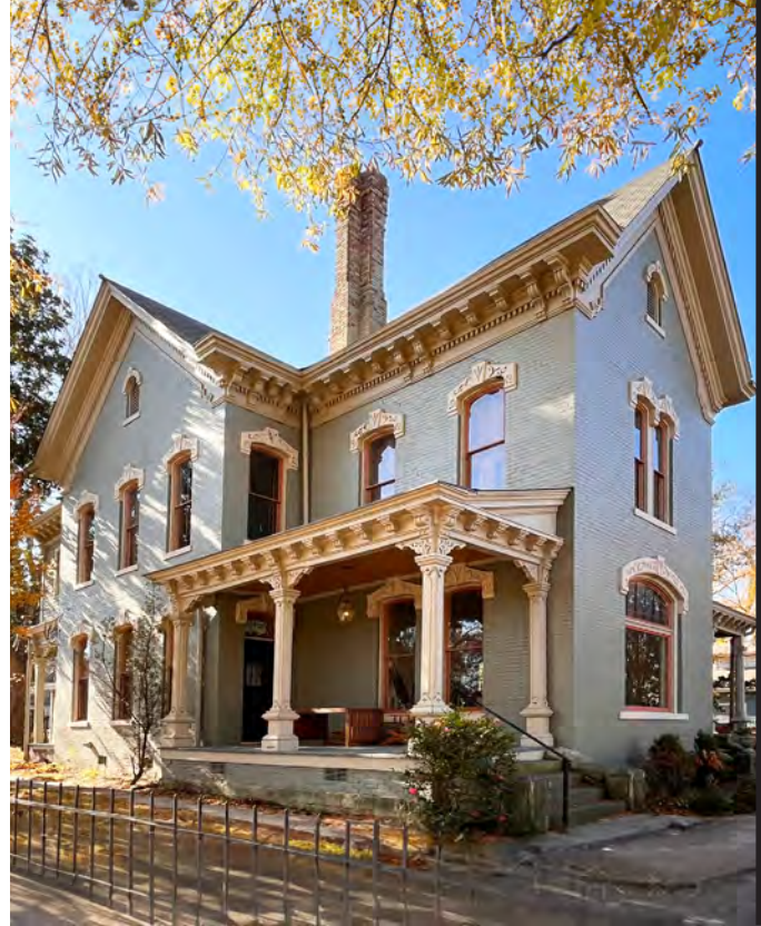
Wood architectural features of the Mills House, 523 E 6th St.
