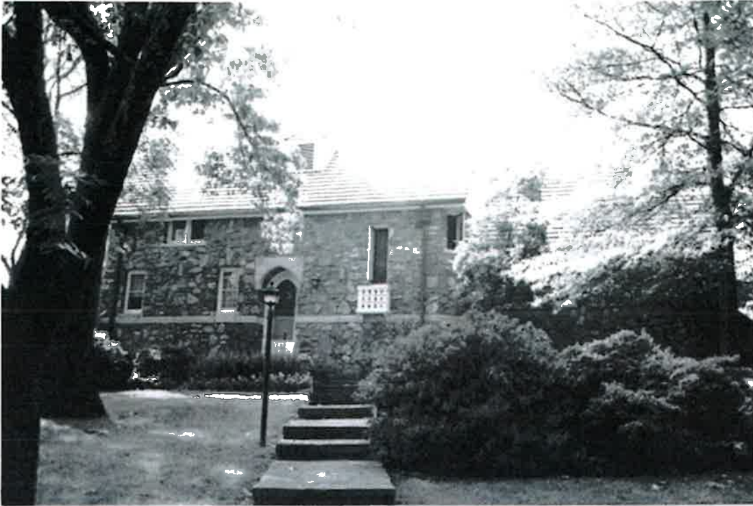
Figure 7: The Holmes House, built in 1928, at 3805 S. Lookout Road in Little Rock, ( image from the 1987 architectural survey in the possession of the Arkansas Historic Preservation Program ).
