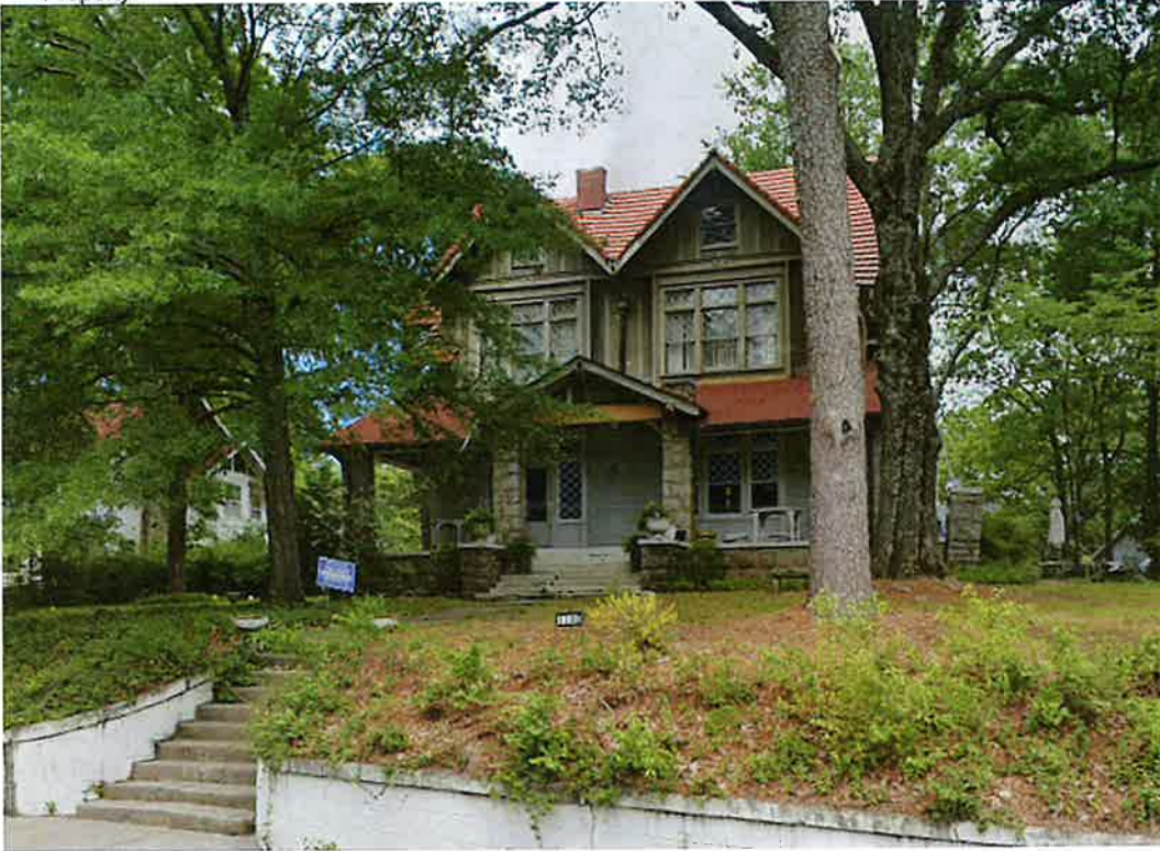
Figure 3: The Volkmer-McKinney House at 1100 Kavanaugh Avenue ( image from the April 2023 Google Street view ).
