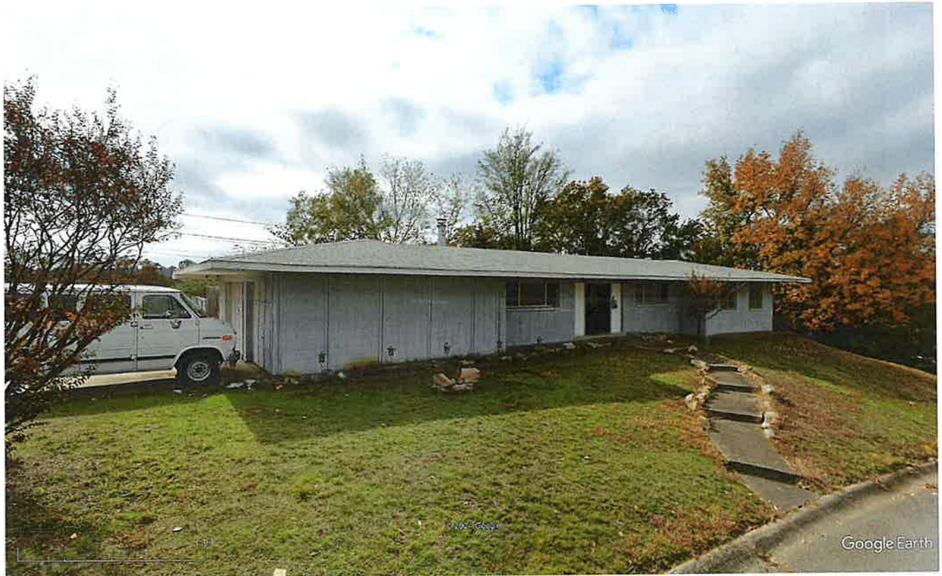
Figure 8: View of John D. Toland and Richard W. Groh Horizon Home from Google Earth, November 2023. The concrete-block screen that originally stood in front of the house has been removed and the carport, which was originally open, has been enclosed into a two-car garage.
