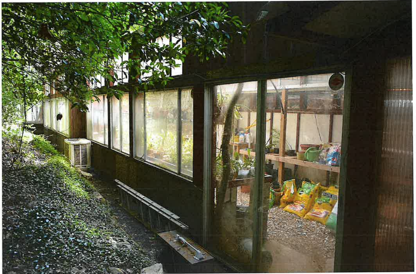
Figure 12: Photo of the rear/northwest façade of the Gibson & Company's Blue Star / Horizon Home prior to the removal of the greenhouse, looking southeast, August 16, 2018.
