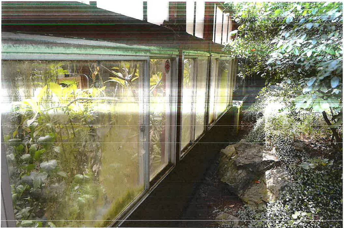
Figure 13: Photo of the rear/northwest façade of the Gibson & Company's Blue Star / Horizon Home prior to the removal of the greenhouse, looking southwest, August 16, 2018.
