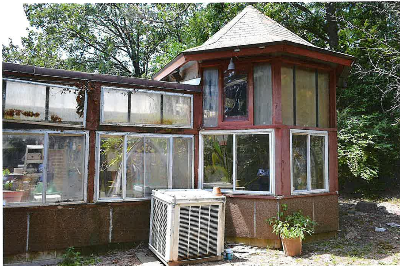
Figure 14: Photo of the side/northeast façade of the Gibson & Company's Blue Star / Horizon Home prior to the removal of the greenhouse, looking northwest, August 16, 2018.
