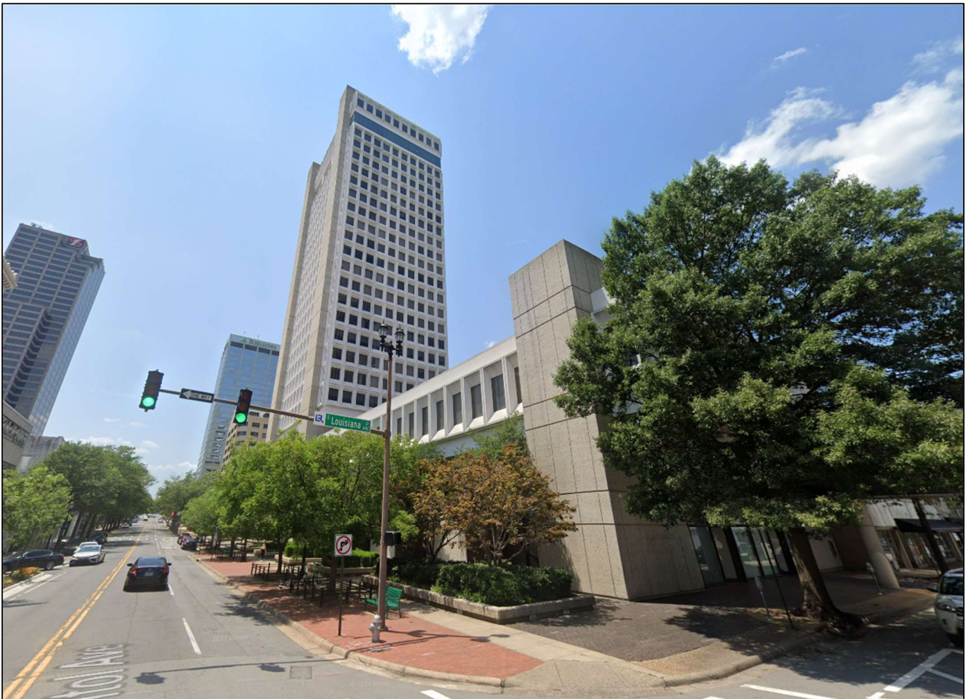
Figure 1. Worthen Building, 200 W Capitol Street, 2023.
