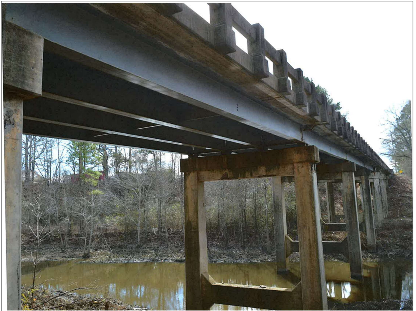
Figure 1. Chicago, Rock Island & Pacific Railway Overpass, 2024.
