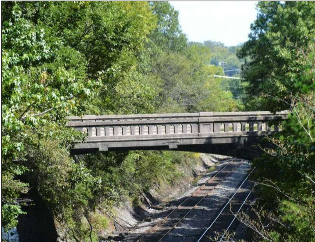
Figure 1. W. 12th Overpass looking north over the railroad tracks.
