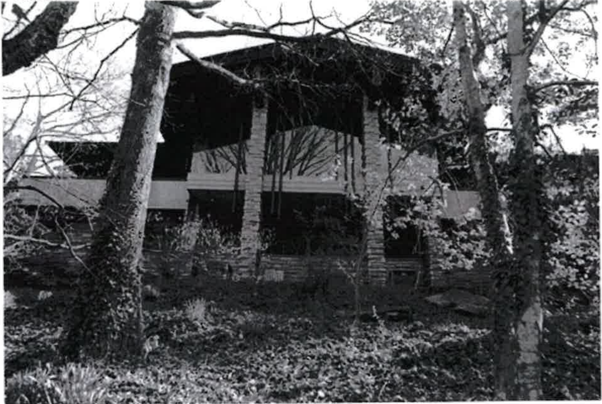
Figure 3: Photograph of the north elevation of the Graham and Louise Hall House (Pine Knoll) from 1999 ( photograph in the survey files of the AHPP ).
