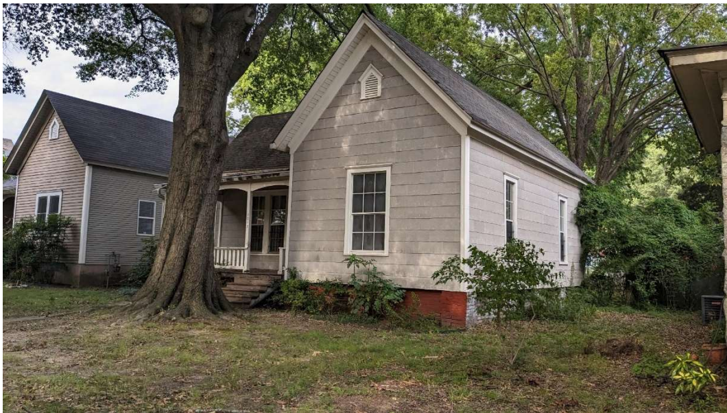
Figure 15. Front facade facing northeast of 1017 S Cumberland.
