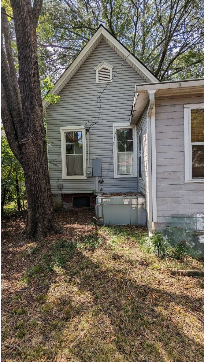
Figure 4. Rear gable of 1017 S. Cumberland.
