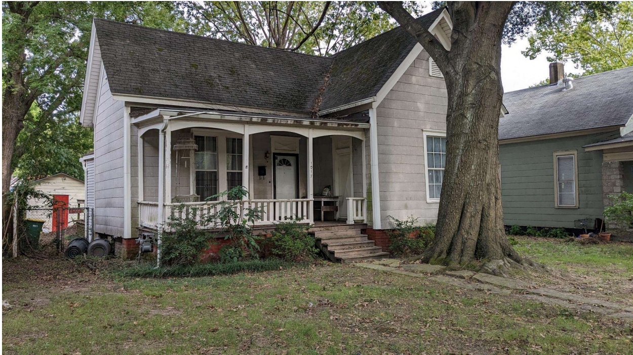
Figure 1. 1017 S Cumberland, front facade, looking east.
