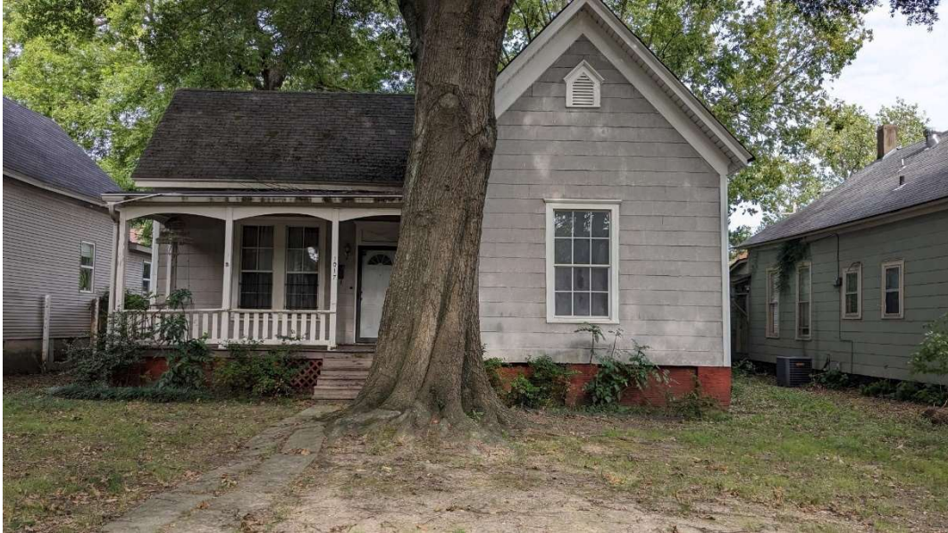
Figure 14. Front facade of 1017 S Cumberland.
