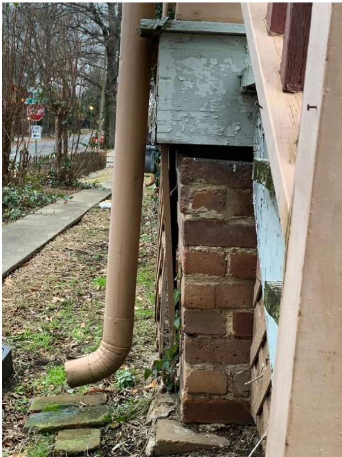
16. NORTH PORCH – NORTHWEST FOUNDATION CORNER
