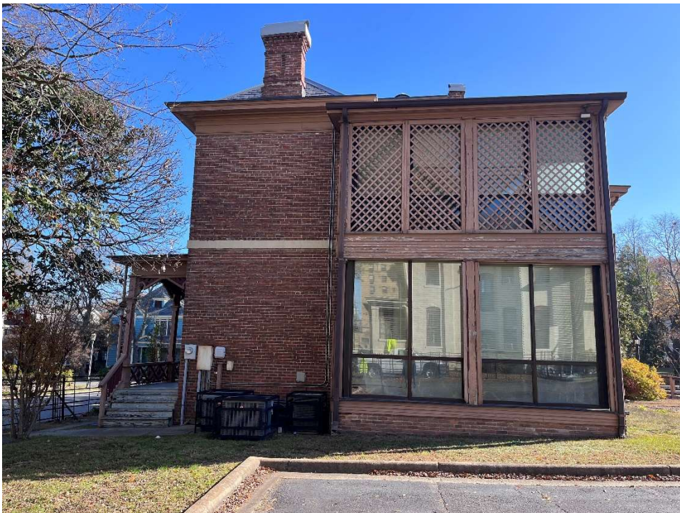
Figure 13. 700 S Rock, west elevation, rear porch, 2023.
