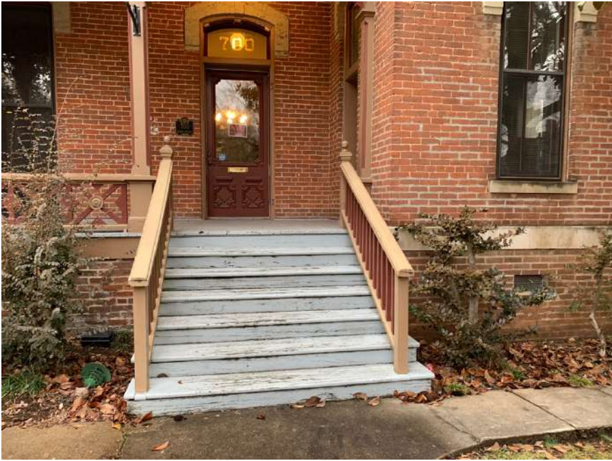
19. FRONT STEPS (EAST FAÇADE)
