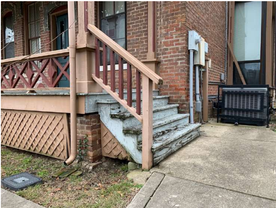
15. NORTH PORCH – NORTHWEST CORNER
