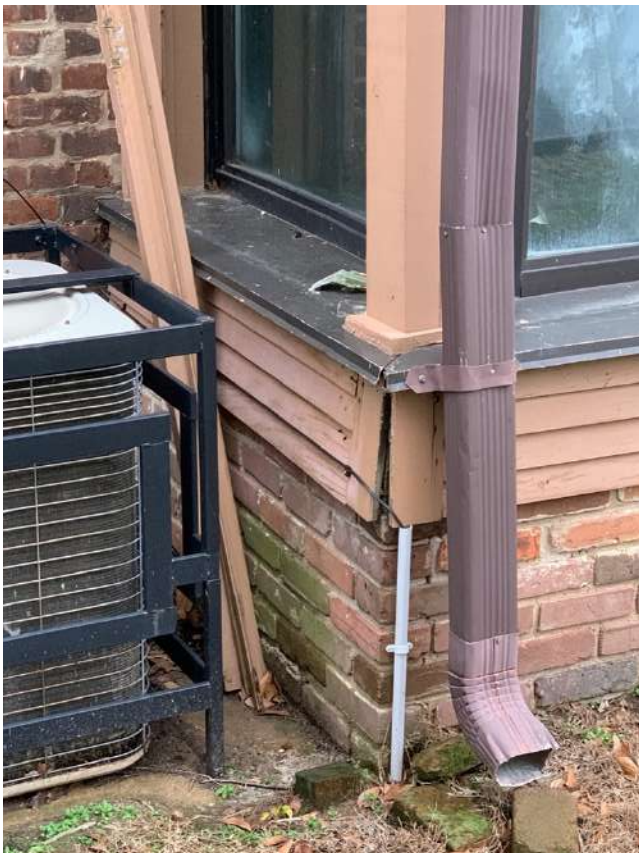
10. WEST PORCH NORTHWEST CORNER
