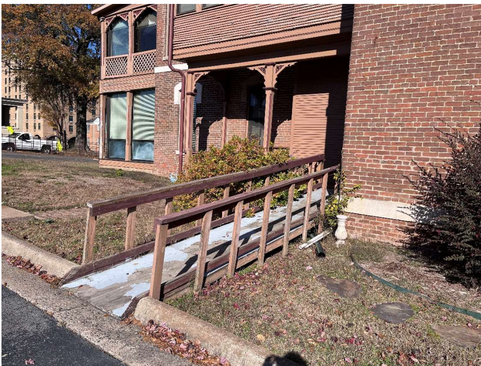
Figure 15. 700 S Rock, south elevation, side porch and existing accessibility ramp 2023.
