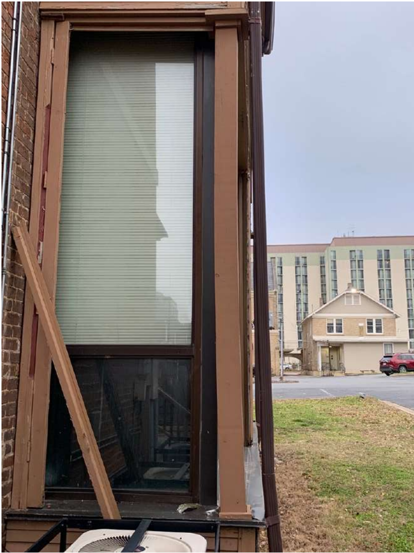
12. WEST PORCH NORTH ELEVATION
