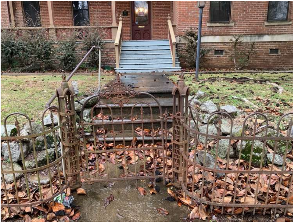
18. EAST (FRONT) GATE AND HANDRAIL
