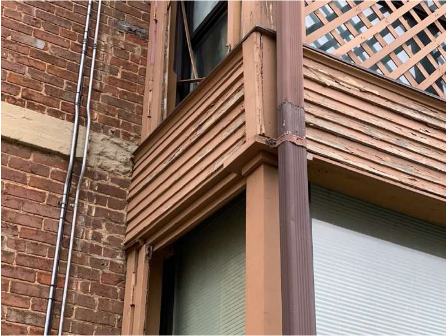
11. WEST PORCH NORTHWEST CORNER
