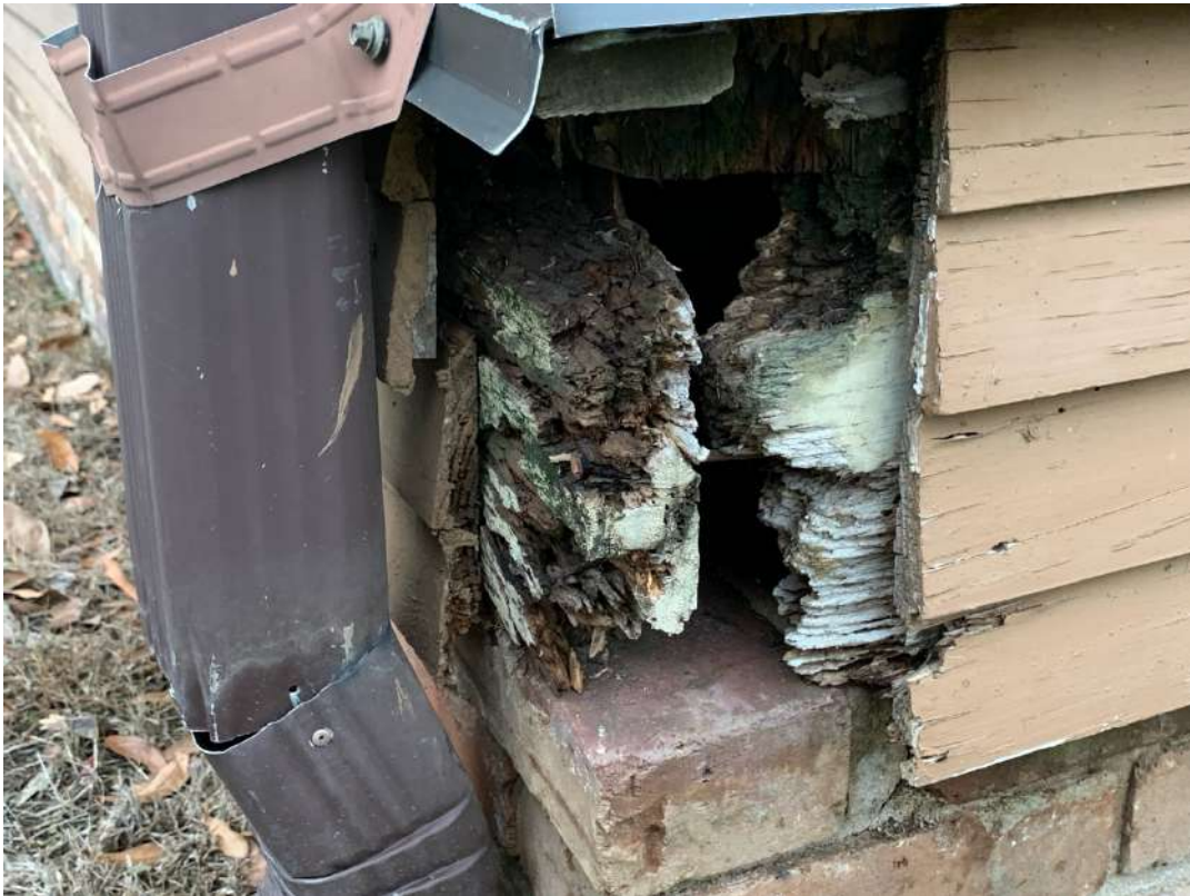
9a. WEST PORCH GRADE BEAM @ SOUTHWEST CORNER
