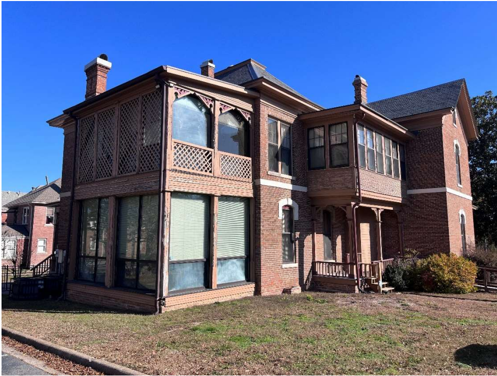
Figure 12. 700 S Rock, south and west elevations, rear porch, 2023.
