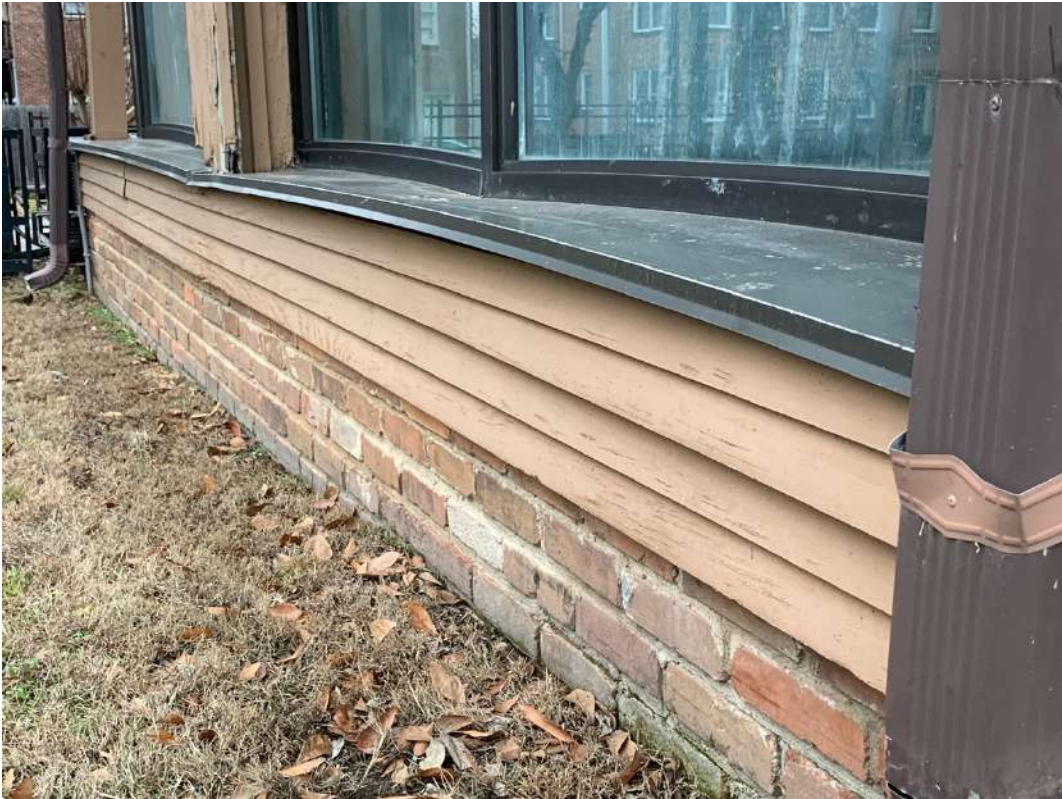
9. WEST PORCH FOUNDATION
