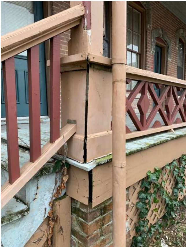
14. NORTH PORCH – NORTHEAST CORNER
