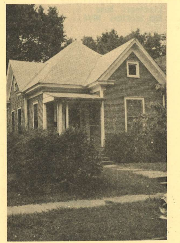
Figure 8. 1420 Commerce front and south facades, looking northwest. Photo from 1978 Quapaw Quarter Architectural Survey.
