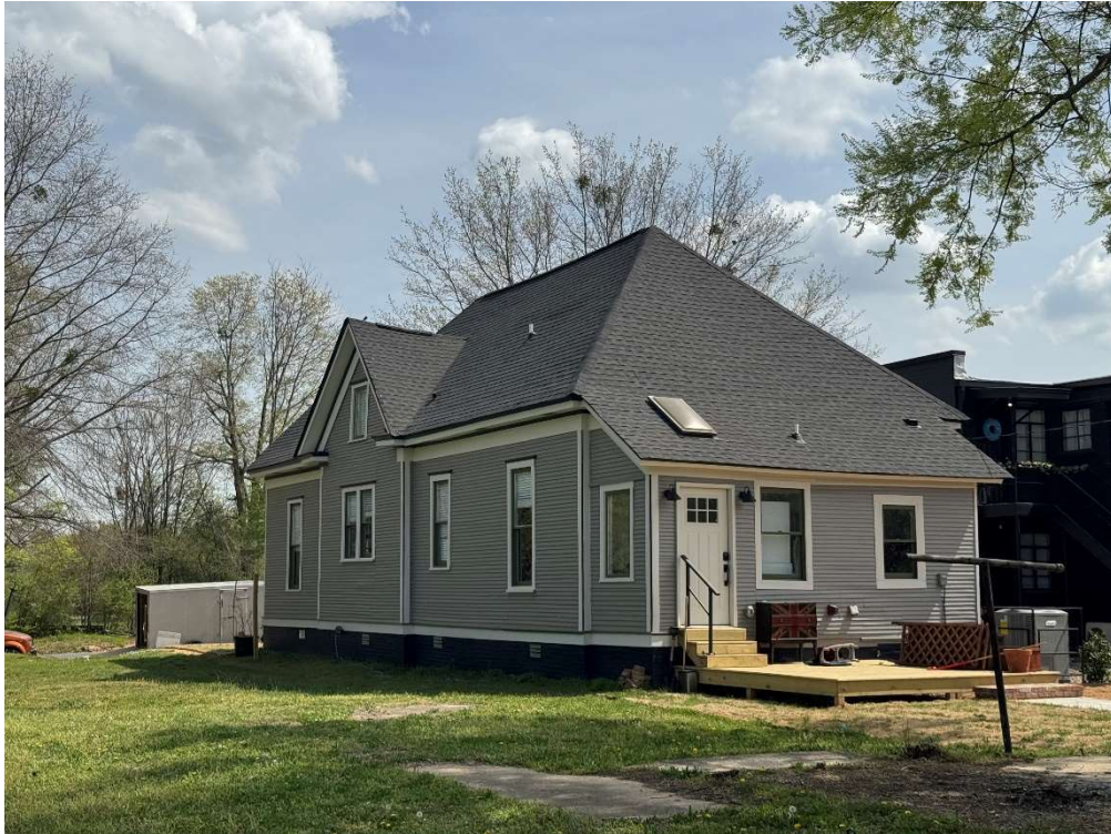
Figure 11. 1420 S. Commerce, west and south elevations, 2025.
