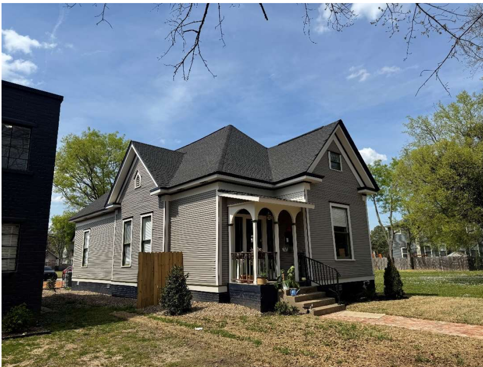
Figure 10. 1420 S. Commerce, east and south elevations, 2025.
