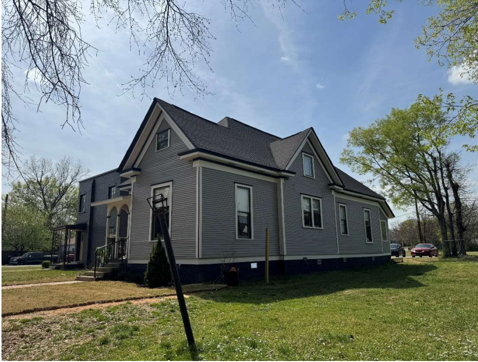
Figure 9. 1420 S. Commerce, east and north elevations, 2025.
