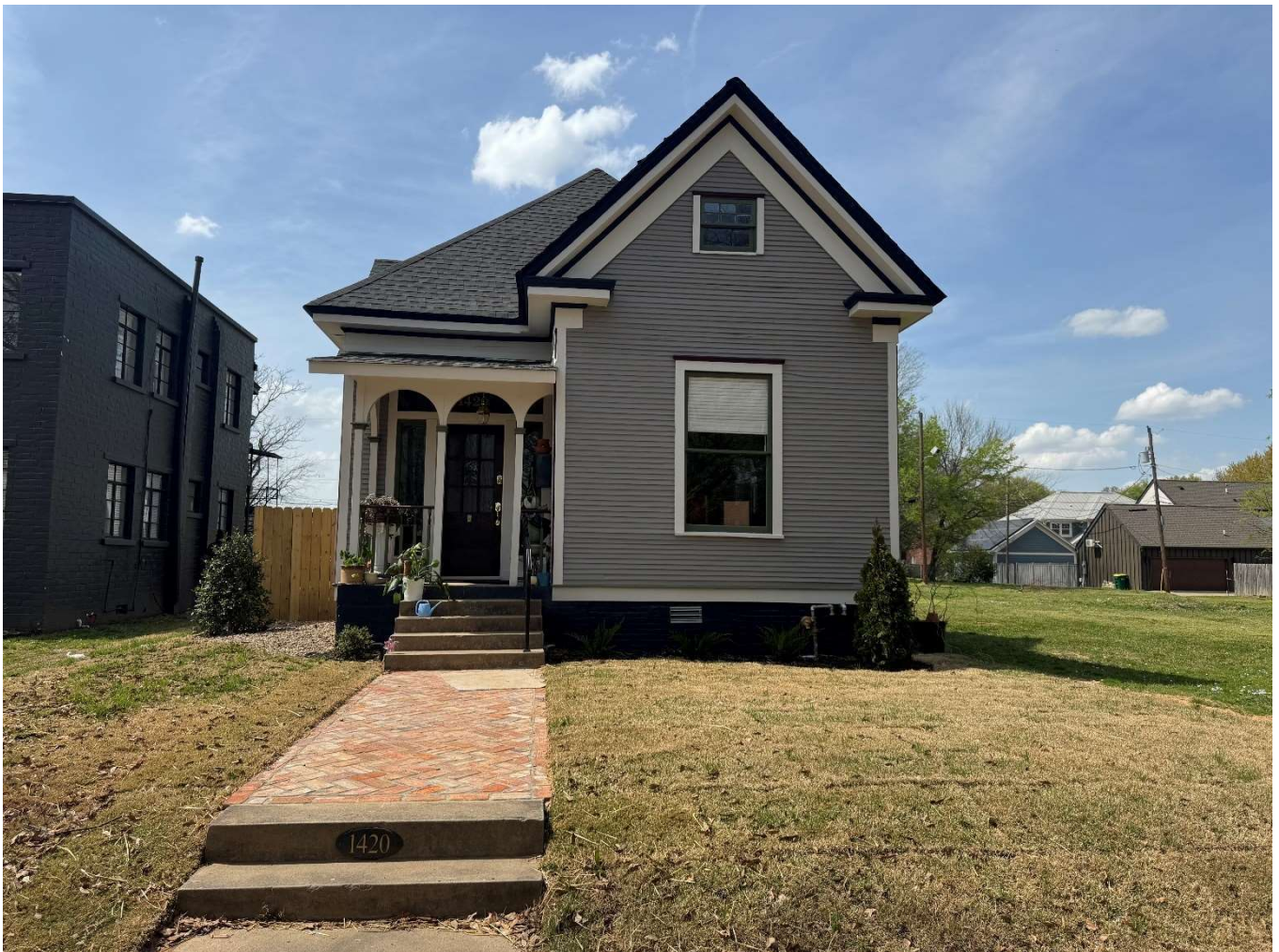
Figure 1. 1420 Commerce Street, Little Rock, 2025.
