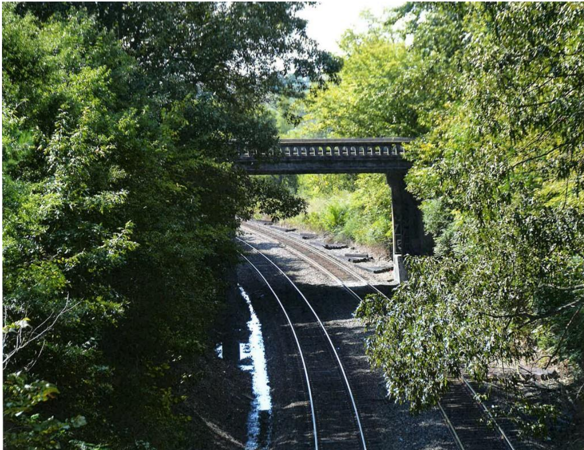
Figure 5. W 14 th Street Overpass, 2024.
