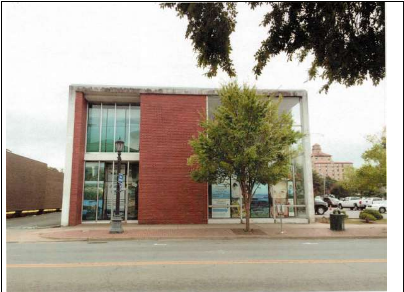
The Paragon Building Existing North Facade 2015
