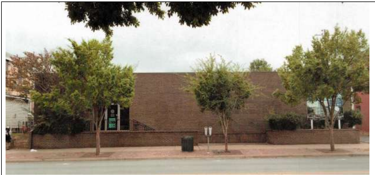
The American Legion Building Existing North Façade 2015
