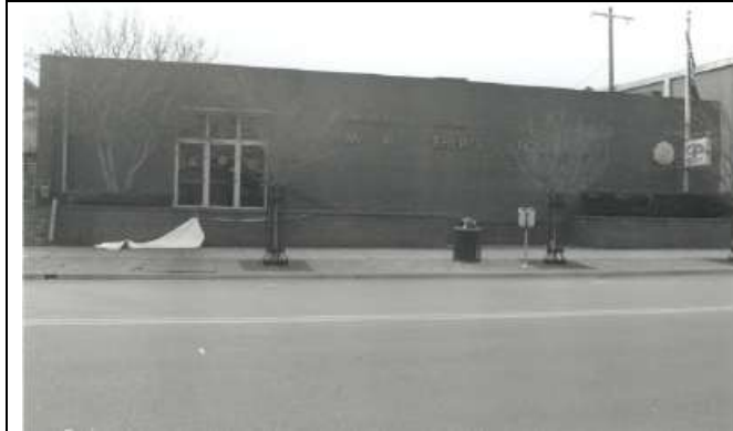
American Legion Building north elevation 2006
