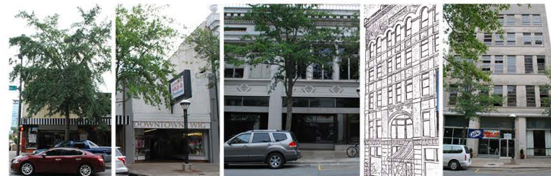
301 Main Street: Menke Building
