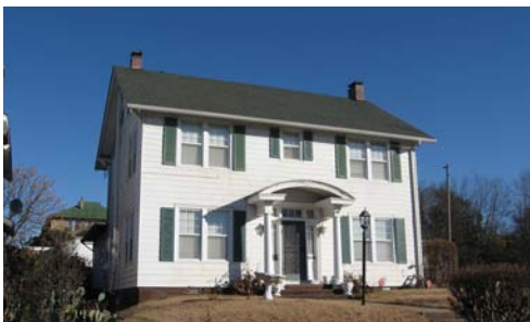
The Historic Preservation Task Force of 1996 stressed the need for completion of survey and National Register efforts for areas such as south of Roosevelt Road (2723 S. Ringo Street).
