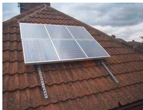
Historic dwellings can be adapted to take advantage of modern energy technology such as solar panels on rear roof lines.
