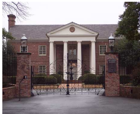
The Governor's Mansion, built in 1950, is one of the focal points of the Governor's Mansion Historic District.
