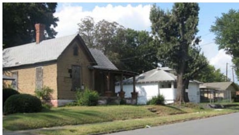
Population loss in the center-city has led to abandoned houses and deteriorated conditions on some blocks such as the 1500 block of S. Pulaski Street....
