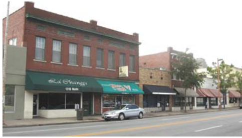
The 1300 block of S. Main Street is part of the Southside Main Street project.
