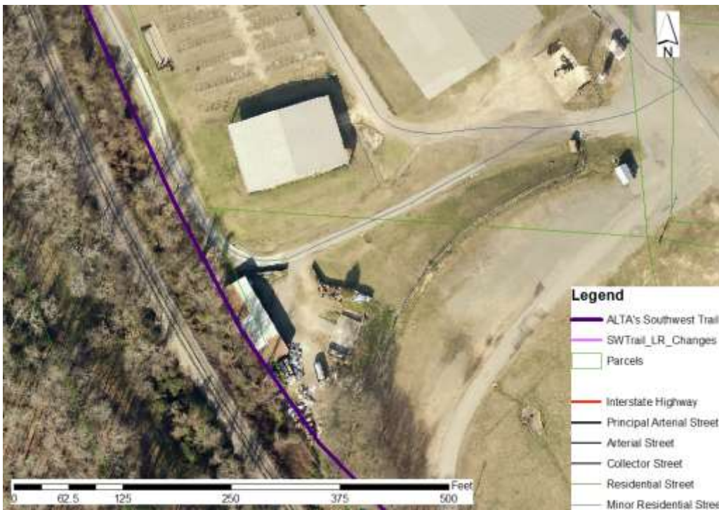
Picture 50. The trail is 63 ft. from active track at its closest point here (going around the building).
