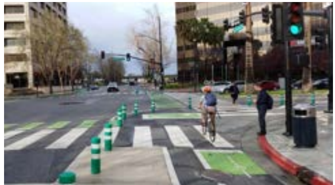
Figure 41: The photo above shows a protected intersection using low cost materials such as plastic bollards and paint.
