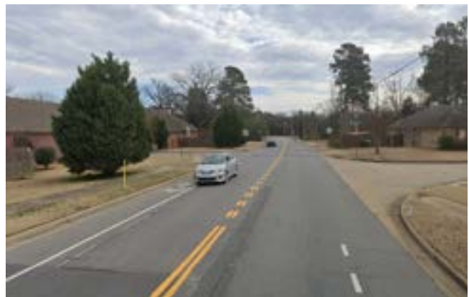
Figure 4: Bike lanes on Taylor Loop Road end before the intersection approach to allow for a left turn lane, leaving bicyclists to merge with traffic and navigate the multi-lane intersection.
