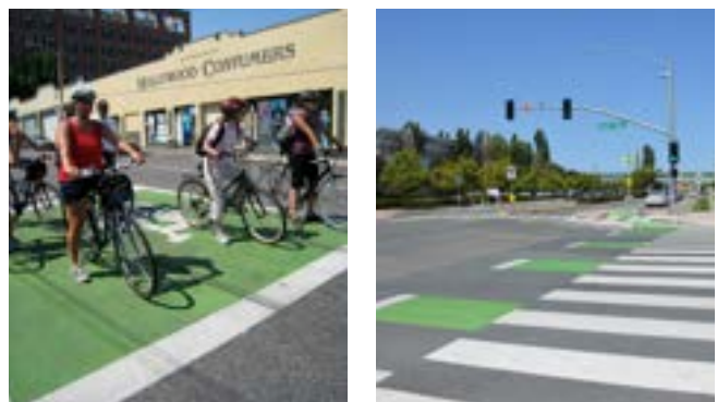
Figure 42: Bike boxes, above left, provide a dedicated space for bicyclists ahead of motor vehicle traffic at signalized intersections. Bicycle crossing markings, above right, provide clear direction for bicycle travel through an intersection.
