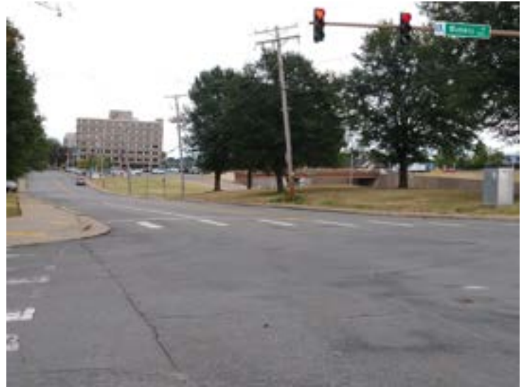
Figure 49: The currently existing four lane cross section on 7th St ends at Battery St. 7th St buffered bike lane configuration should continue to Battery St (and further west), which is a key north/south crossing for bicyclists of I-630.
