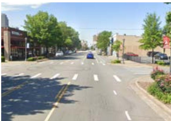
Figure 57: S. Main St from 7th St in downtown to Roosevelt Rd was reconfigured from four lanes to three with the creation of bike lanes in 2013 as part of a resurfacing project. 'Pop in the Rock', an annual tactical urbanism event created by studioMain was a key reason for the Main St transformation.
