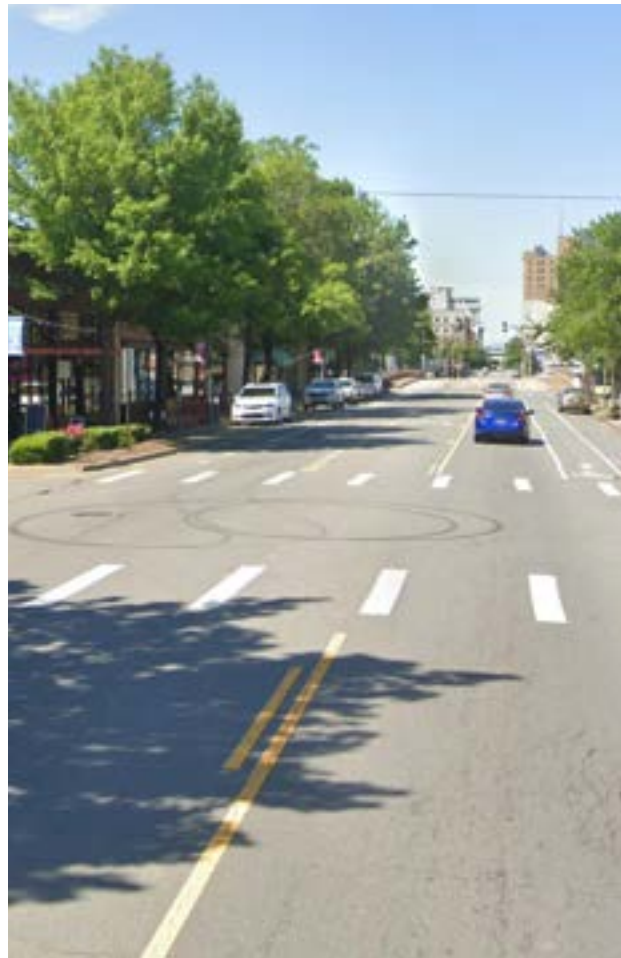
Figure 63: S. Main St from 7th St in downtown to Roosevelt Rd was reconfigured from four lanes to three with the creation of bike lanes in 2013 as part of a resurfacing project. 'Pop in the Rock', an annual tactical urbanism event created by StudioMain was a key reason for the Main St transformation.
