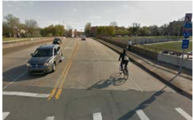
Figure 3: Buffered bike lanes on South Main Street over Interstate 630.
