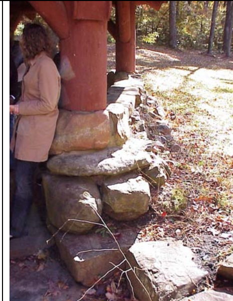
A Pier of the Springhouse.
