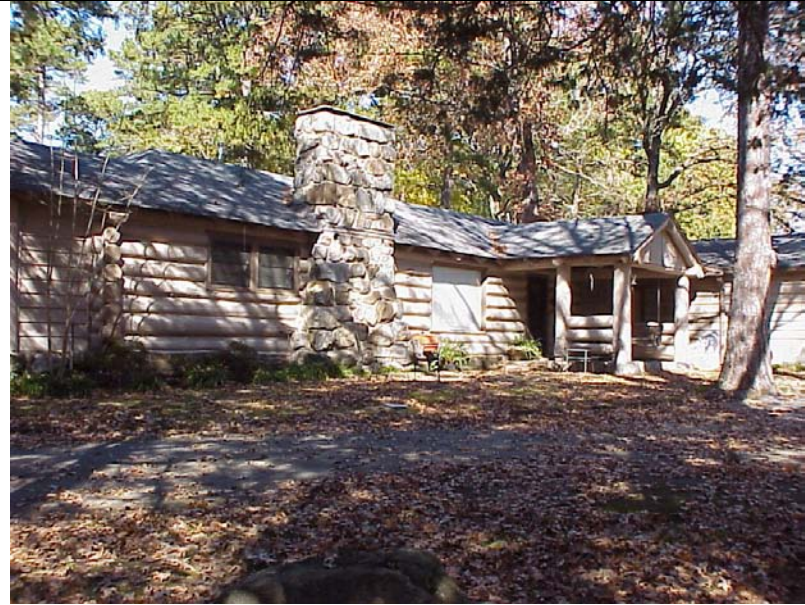
Caretaker's cabin rear façade from south showing addition of gabled porch and garage to the right.
