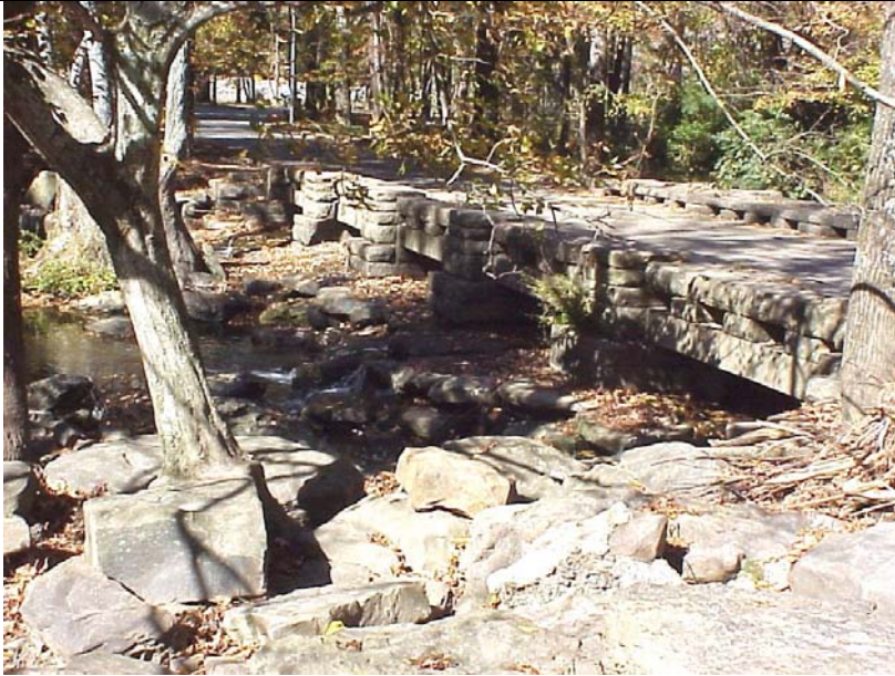
South elevation of low water bridge.
