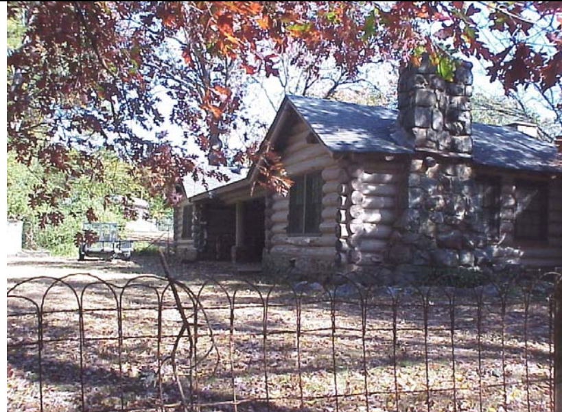
Caretaker's cabin front façade from south.
