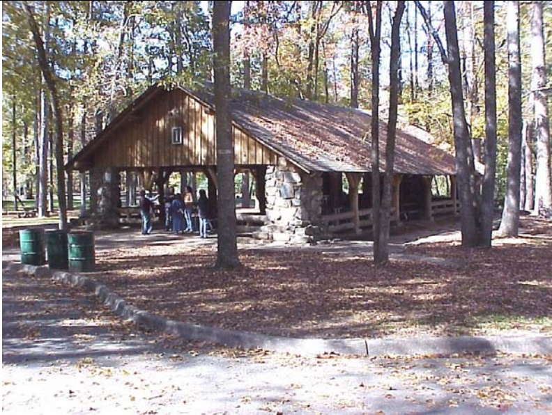
Pavilion #1 from the east.
