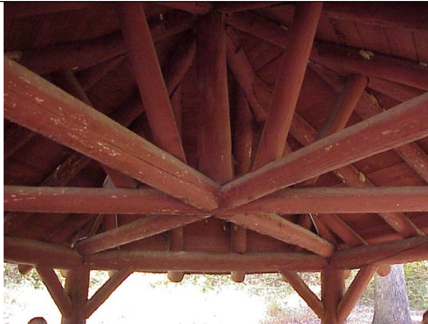
Interior beams of the Springhouse.
