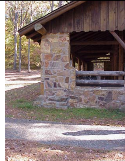
Corner detail of Pavilion #2
